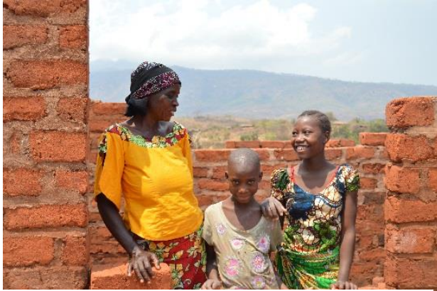
Mama Shukrani Shaban, a Model Household motivator trainee with her daughters in front of their new house under construction in Buhingu. Photo Credit: Nelson Mmari, TNC
